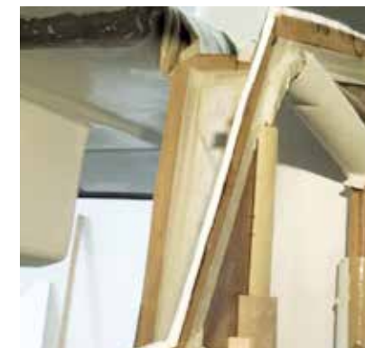
Fig. 92 Sikaflex®-292i applied to a lightweight panel prior to fitting
