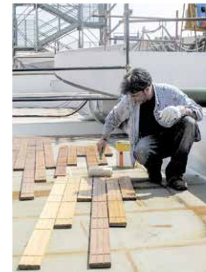
Fig. 35 Applying Sika® Primer-290 DC or Sika® MultiPrimer Marine to a teak deck with a roller (hidden side)
