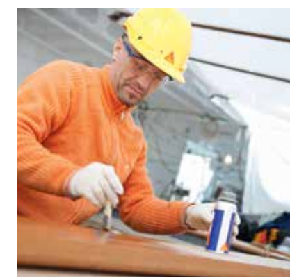
Fig. 36 Carefully applying Sika® Primer-290 DC or Sika® MultiPrimer Marine
