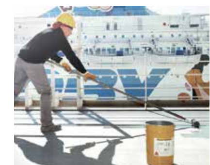
Fig. 29 Applying SikaCor® ZP Primer with a roller
