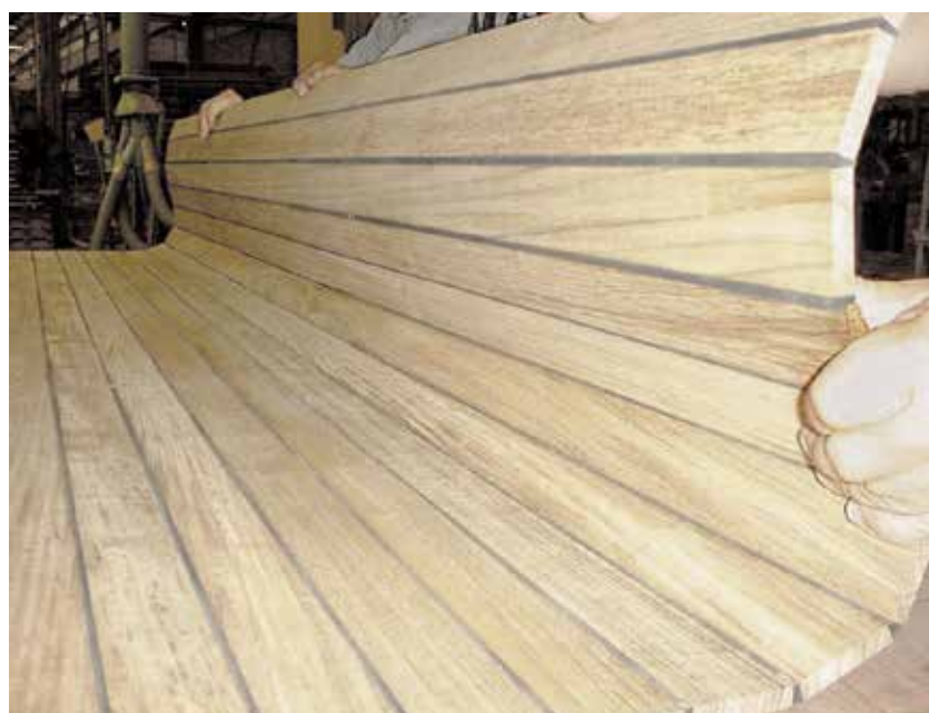
Fig. 49 Deep joint prefabricated teak decking and the strength and flexibility inherent in the adhesive
