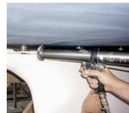
Fig. 106 The adhesive is applied
