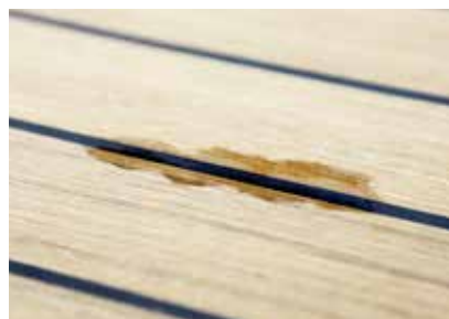
Fig. 58 Discolouration of the wood is a tell-tale sign of a failed or damaged joint in this teak deck
