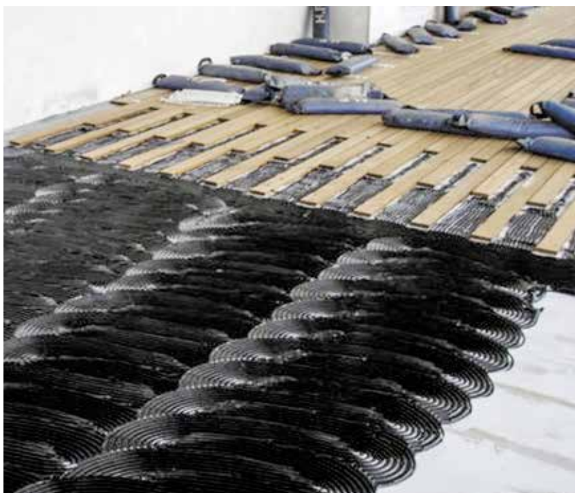
Fig. 40 A teak floor being laid, showing the bedding compound and the weights to hold it in place
