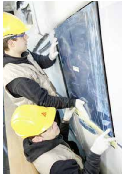
Fig. 101 The window is fitted
