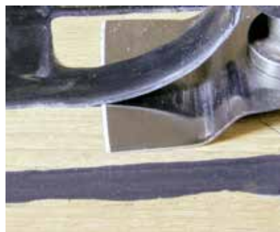
Fig. 75 Picture Removal overstanding Sikaflex®-290 DC PRO with a vibrating scraper power tool
