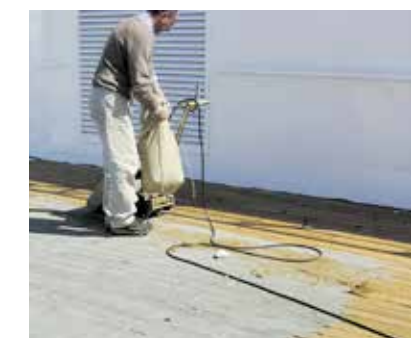
Fig. 46 Sanding the deck
