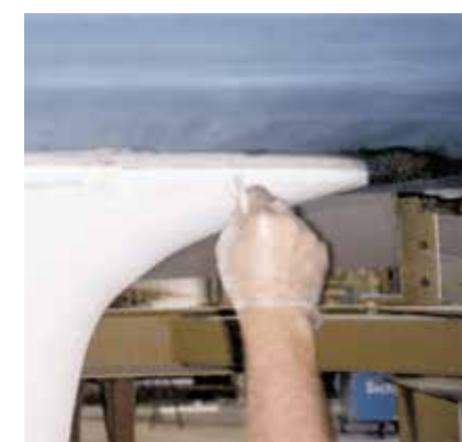
Fig. 107 The joint is tooled off and finished
