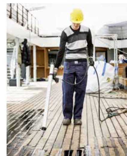
Fig. 43 Applying Sikaflex®-290 DC PRO
