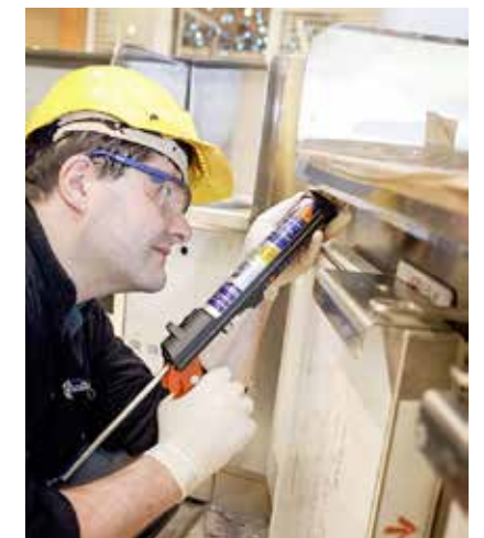
Fig. 90 Application of Sikaflex®-291i
