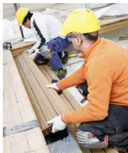
Fig. 39 Putting down the decking
