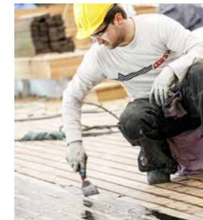
Fig. 45 Compressing Sikaflex®-290 DC PRO with a spatula
