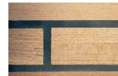
Fig. 55 New teak deck
