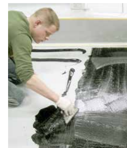
Fig. 81 Application of Sikaflex®-298
