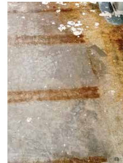
Fig. 28 Typical welds and weld splatter of a steel deck
